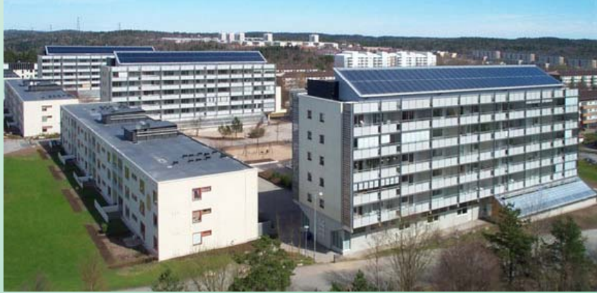
Gardsten, Sweden Three 7 storeys buildings, around 1970 Each 240 m 2 solar collectors + 20 m 3 storage
