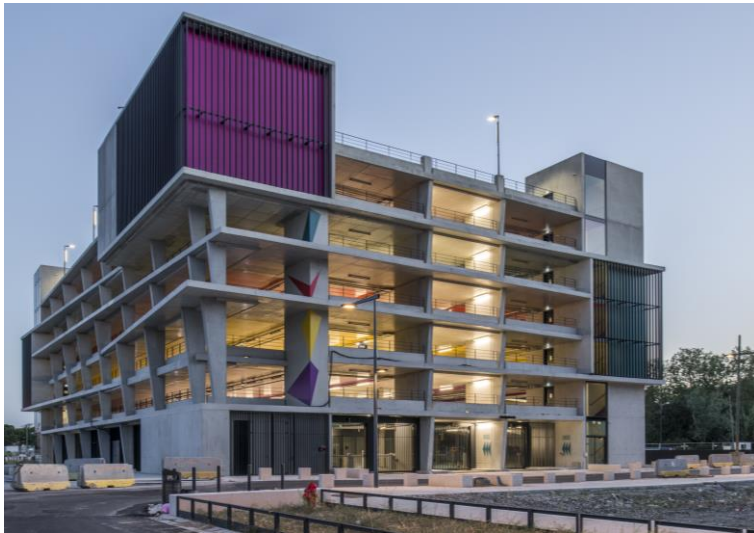
Parking public en silo (Toulouse)
