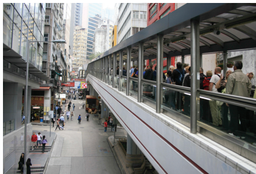
Escalator roulant, Hong Kong
