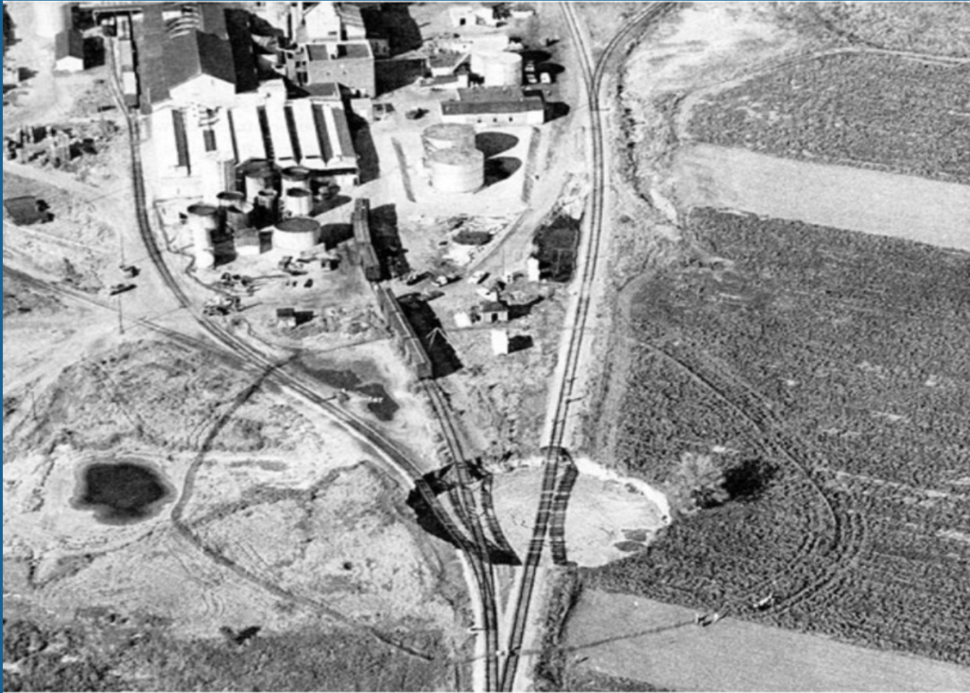
Cargill salt plant, Hutchinson, Kansas, 1974. Some 14 hrs after the collapse, the sinkhole diameter was 200 ft. (Photograph by Hutchinson News , October 21, 1974.)
